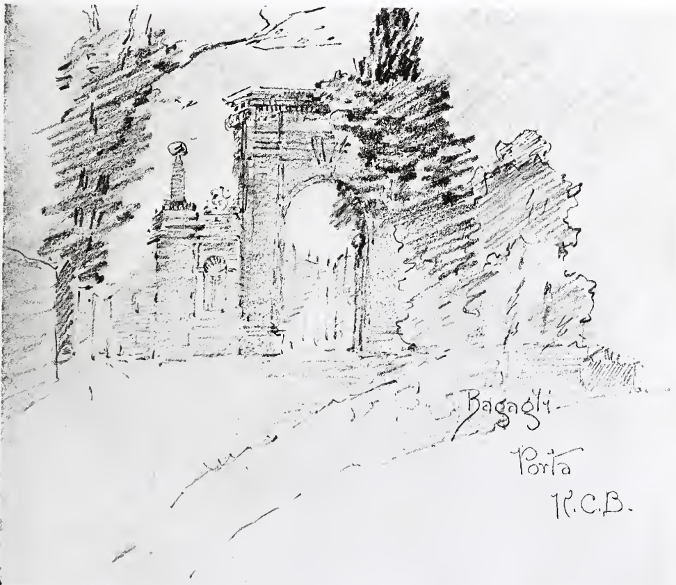
THE RENAISSANCE GATE LEADING TO THE BAGAGLI VILLA.
